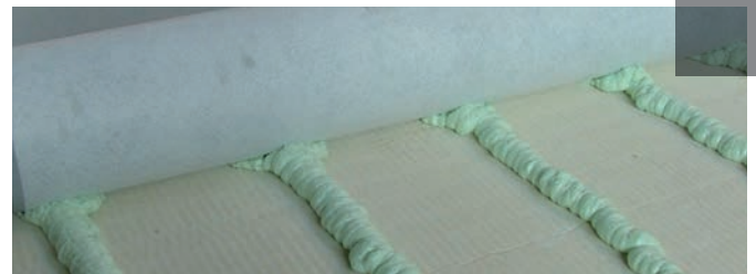
A bonded membrane incorporating HARDROCK® Multi-Fix (DD)
